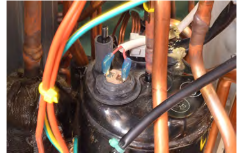
Compressor Overload
