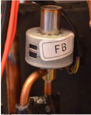
Electronic Expansion Valve
