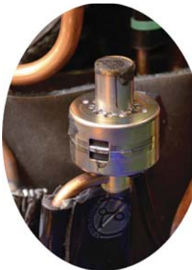
Electronic Expansion Valve
